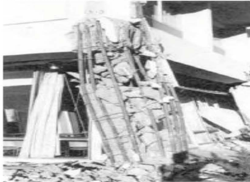
(b) Brittle failure of a reinforced concrete column
