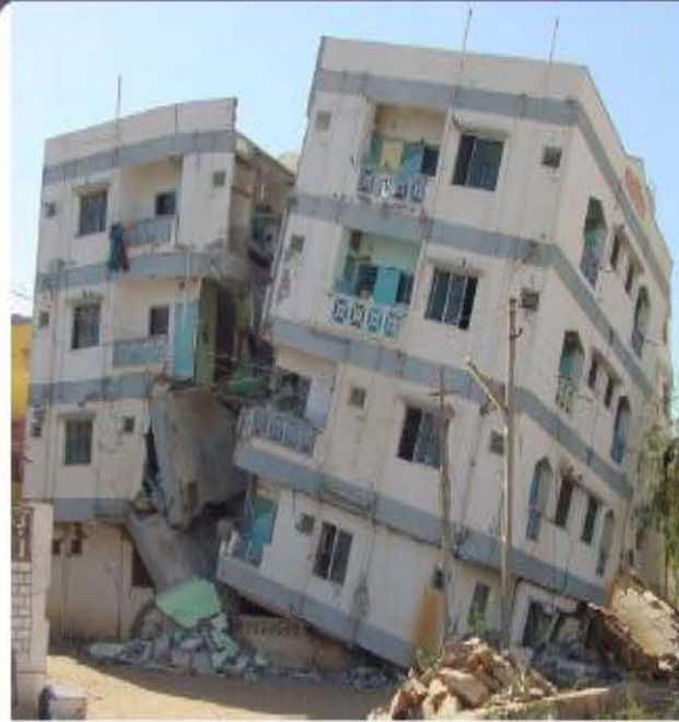
Figure 1: Total horizontal earthquake force in a building increases downwards along its height.
