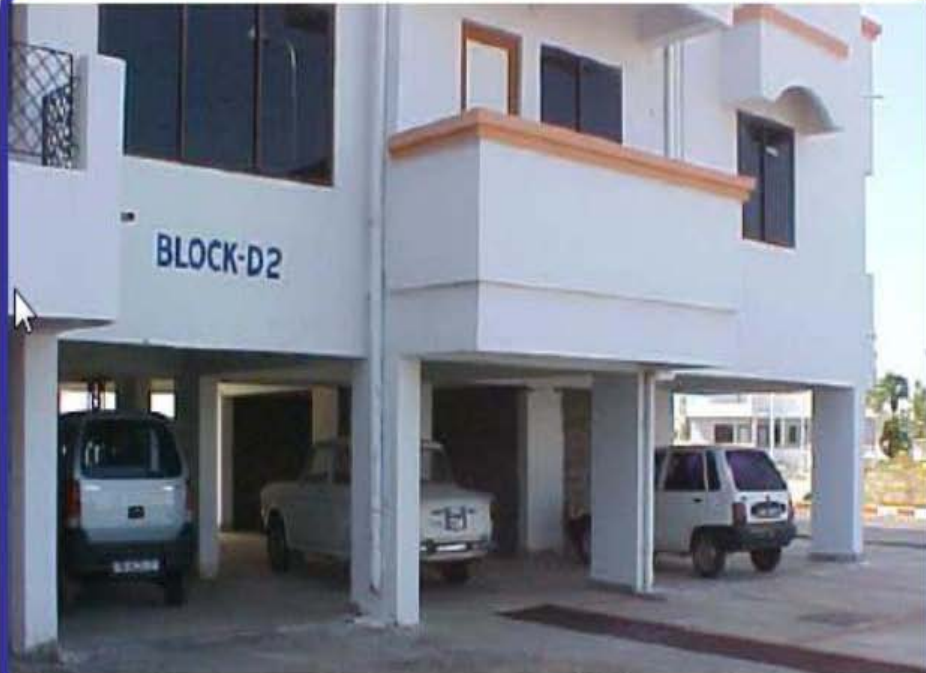
Figure 1: Ground storeys of reinforced concrete buildings are left open to facilitate parking – this is common in urban areas in India.
